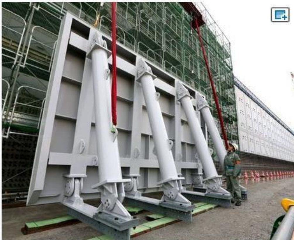
A four-meter-tall steel plate is moved into position to raise the height of the breakwater at the Hamaoka nuclear power plant in Omaezaki, Shizuoka Prefecture, on Dec. 19. (Yoichi Kawatsu)
