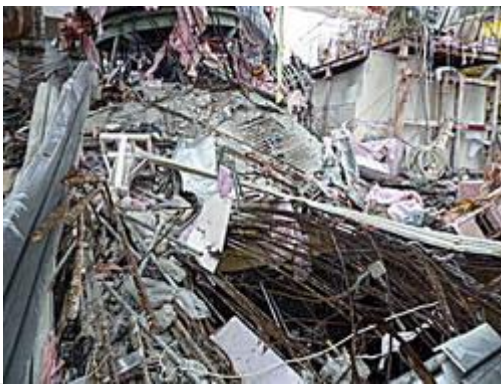
The fifth floor of the No. 4 reactor building at the Fukushima No. 1 nuclear plant is seen with its floor ballooned upward. (Photo courtesy of TEPCO)
